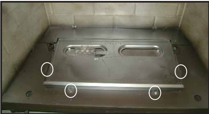
Figure 3.9 Remove Burner Skirt
