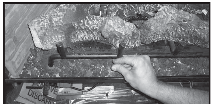
Figure 14.4 Placement of Vermiculite
