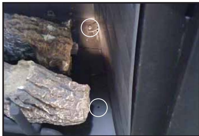
Figure 3.5 Bottom Screws For Metal Refractory
