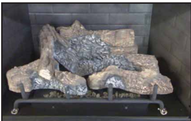
Figure 3. Left Log in Proper Position
