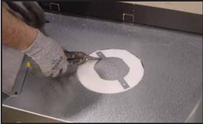
Figure 9.1 Cut the seal cap strap across the rectangles next to the disk. For rear vent, skip this step.
