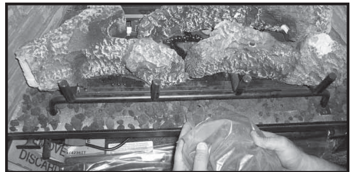
Figure 14.3 Placement of Lava Rock
