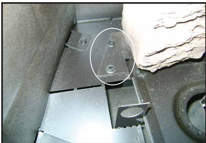
Figure 3.4 Remove Screws from Log Tabs
