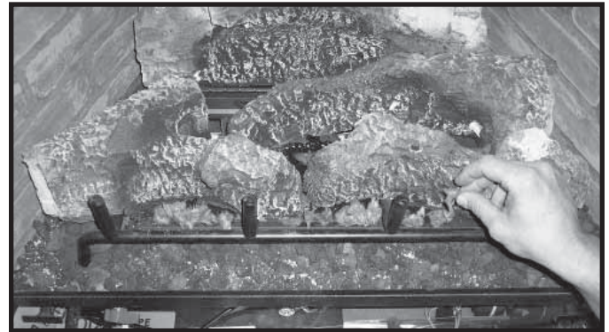
Figure 14.1 Placement of Embers
