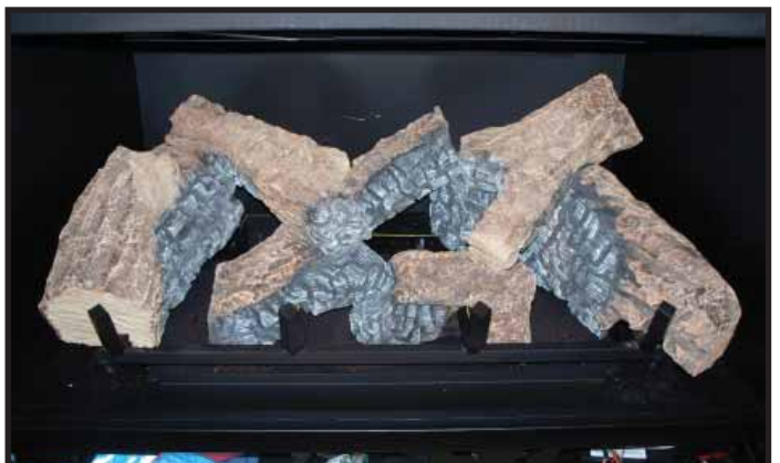
Figure 9. Log Set Installed
