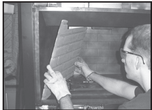
Figure 4 - Tip Side Refractory
