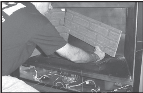
Figure 7 - Place Back Refractory-B-Vent
