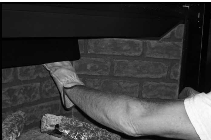
Figure 9 Set Side Refractory in Place
