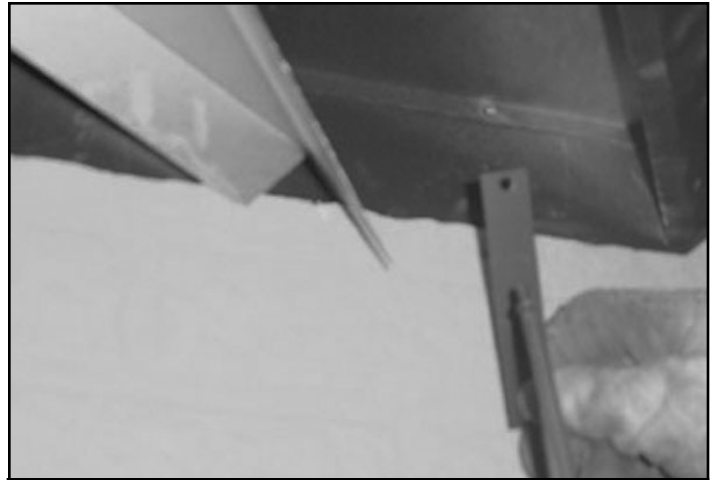
Figure 10 Attach Refractory Bracket
