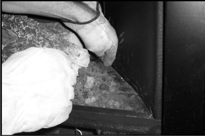
Figure 7 Move Lava Rock to Install Side Refractory
