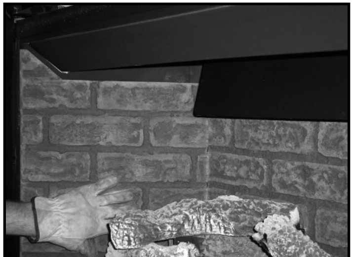
Figure 11 Install Other Side Refractory
