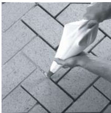
Figure 25 - Grouting Brick
