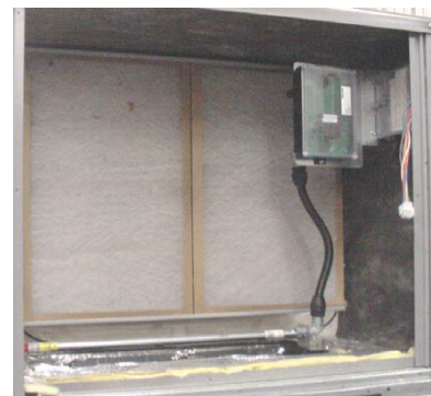
Fig. 64 - Return Air Sensor Operating Position
