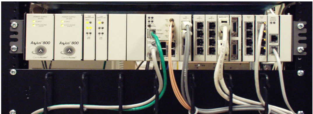
Axxius 800 mounted to a 19" rack with mounting brackets
