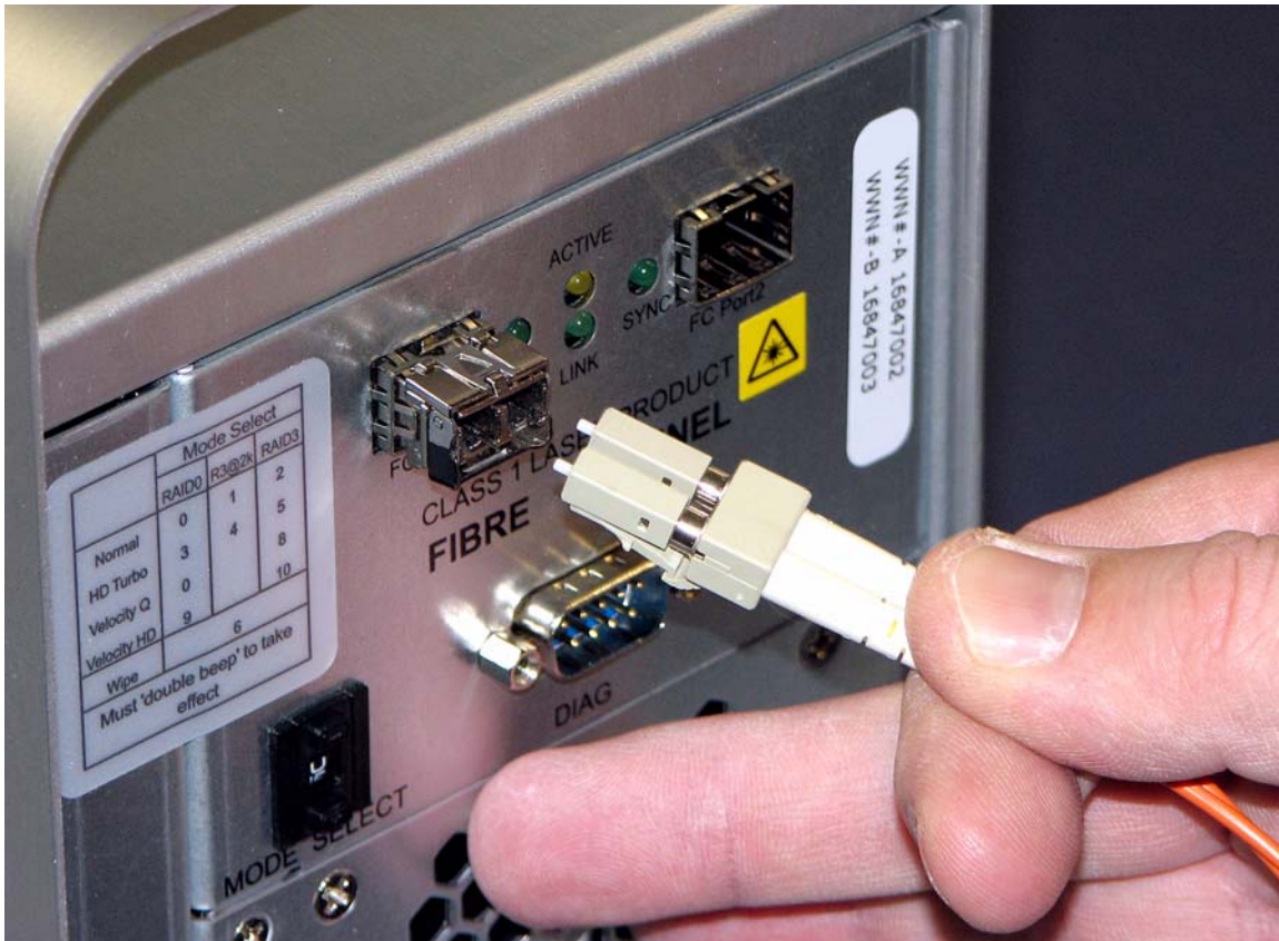
FIGURE 4-4. LC Duplex Cable Being Inserted into the SFP (at FC Port 1).
