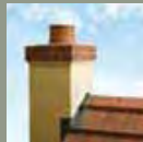
Brick/Stone Chimney (Class 1) 1
